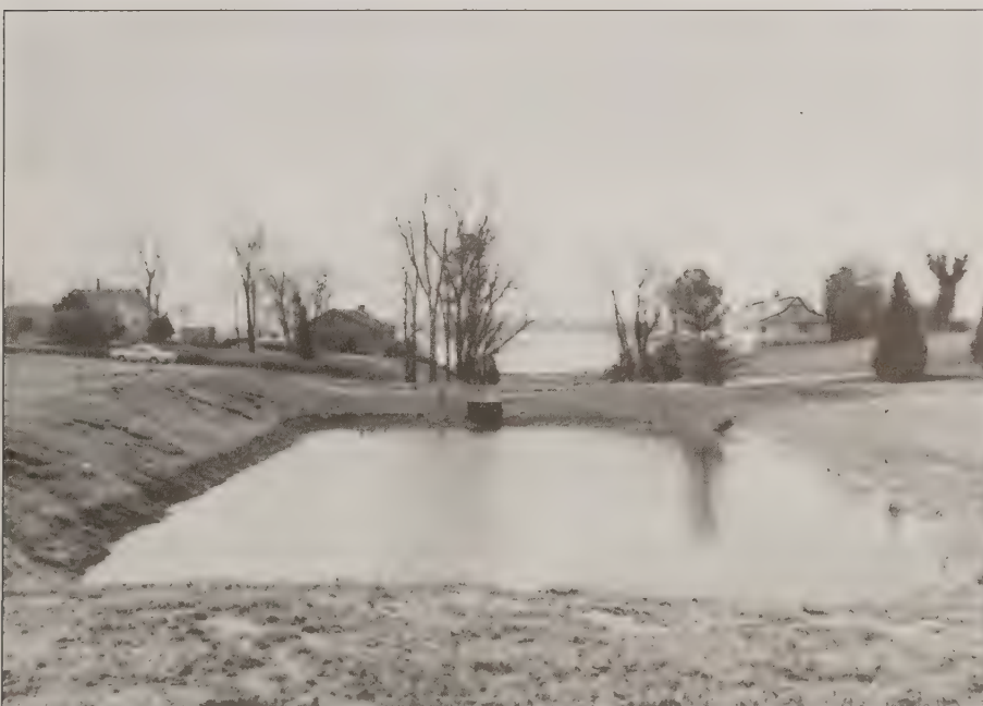
Sediment Control Pond
